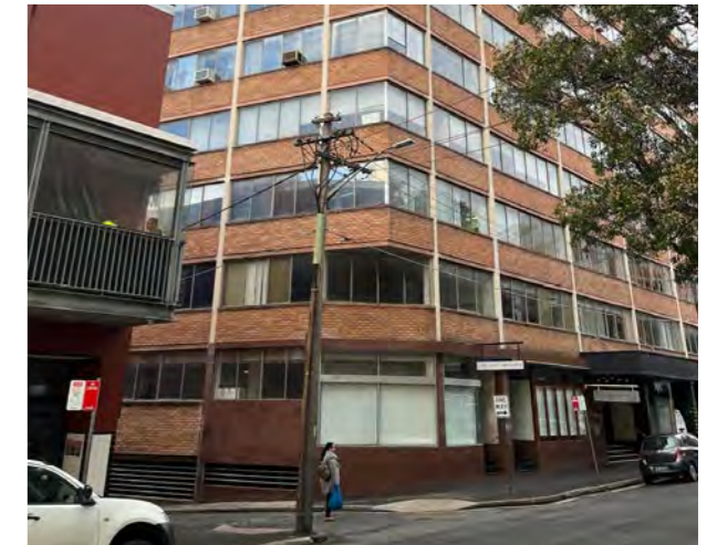
View 6. Looking east along Kippax Street
