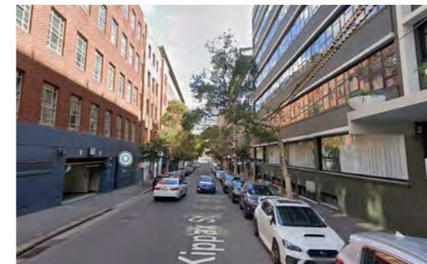
5. Bulk and Massing View from Kippax St
