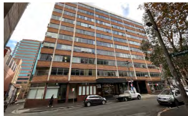
View 1. Looking north east at corner of O'Loughlin and Kippax Street
