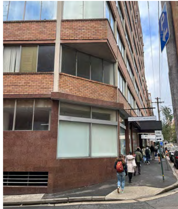
View 7. Looking south east at corner of Terry and Kippax Street
