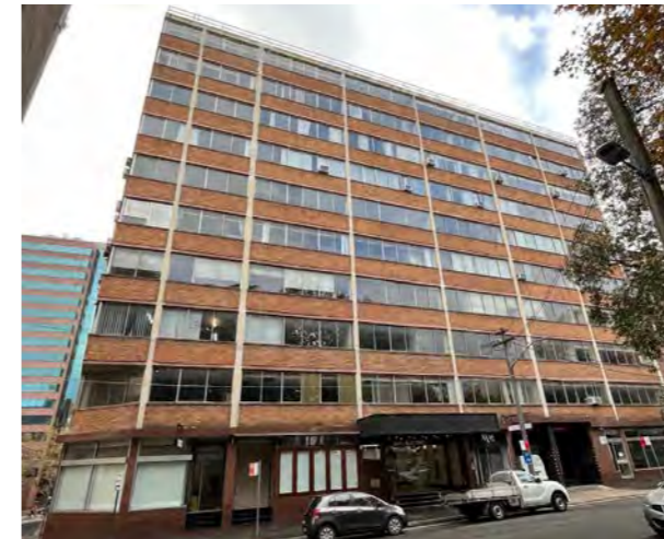
View 5. Looking north east at corner of O'Loughlin and Kippax Street
